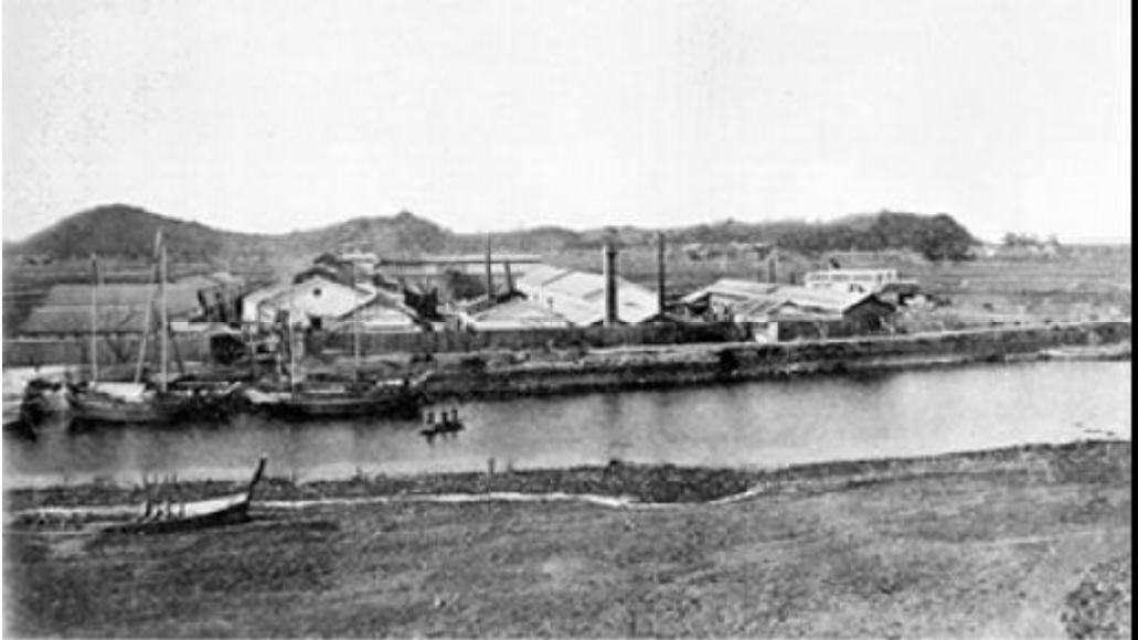
The old Chisso factory constructed in the Meiji period
